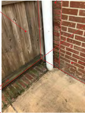
3 VIEW FROM ARCHIBALD WALK LOOKING SE
