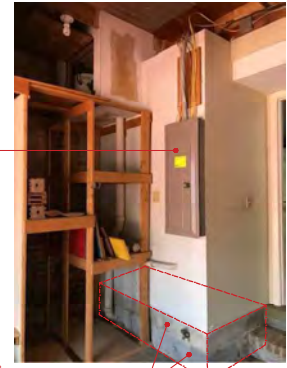
4 GARAGE INTERIOR / SLAB TRANSITION
