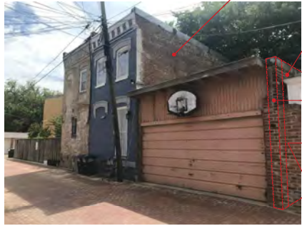
2 VIEW FROM ALLEY LOOKING SW
