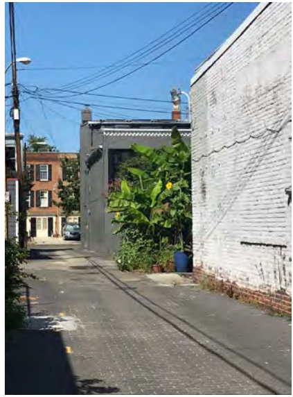
3. View of parapet of dwelling from Archibald walk
