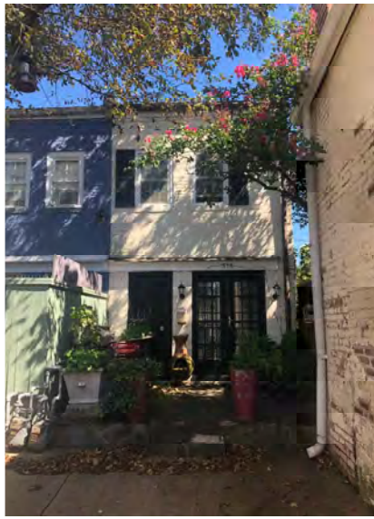
2. View of adjacent dwellings
