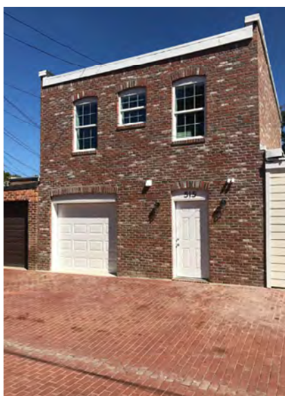
5. Structure opposite Garage
