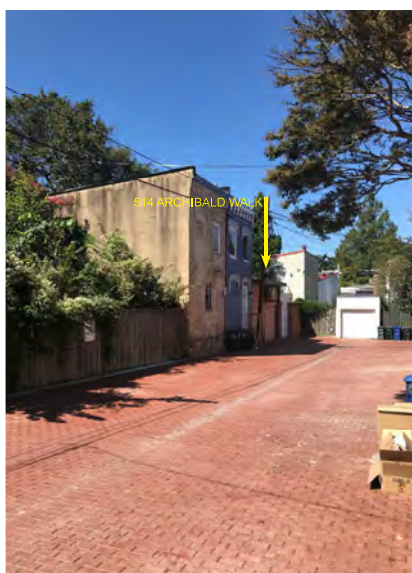
6. View of Public Alley
